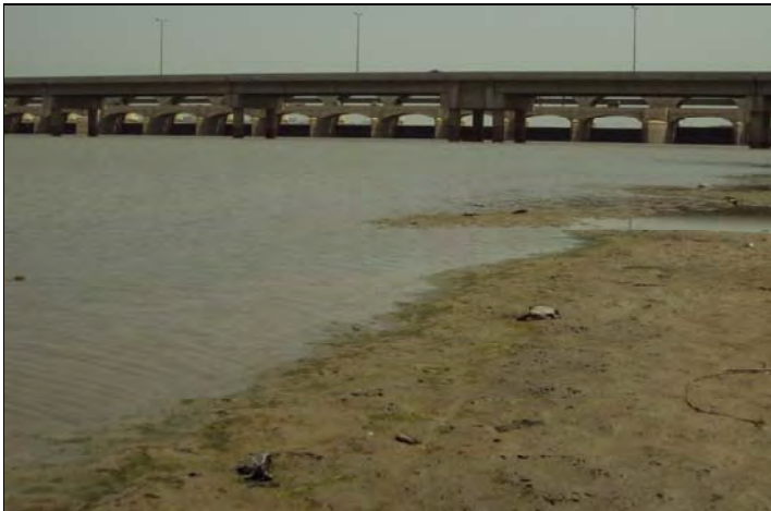
Downstream Sukkur Barrage, the Indus River
